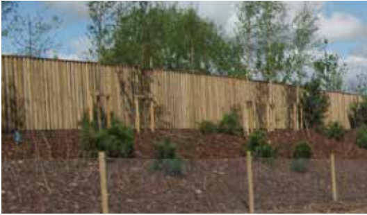
Acoustic fence to a perimeter mounds where applicable
