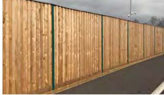
Typical Acoustic Fencing
